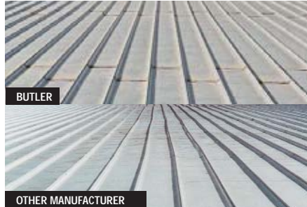
Above Top: Butler's factory punching assures straight panel alignment.
