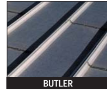
Above Bottom: Without factory punching, these misaligned panels bind on clips, strain seams and compromise weathertightness.
